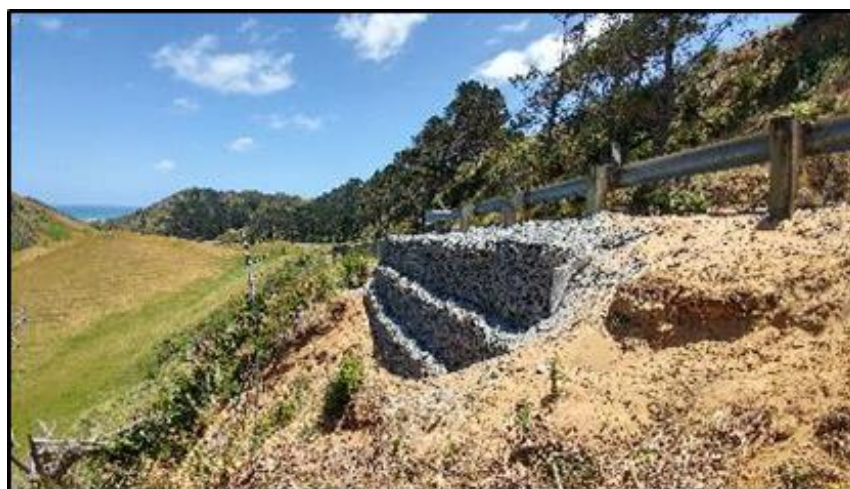
New gabion wall - Glinks Road underslip repair
