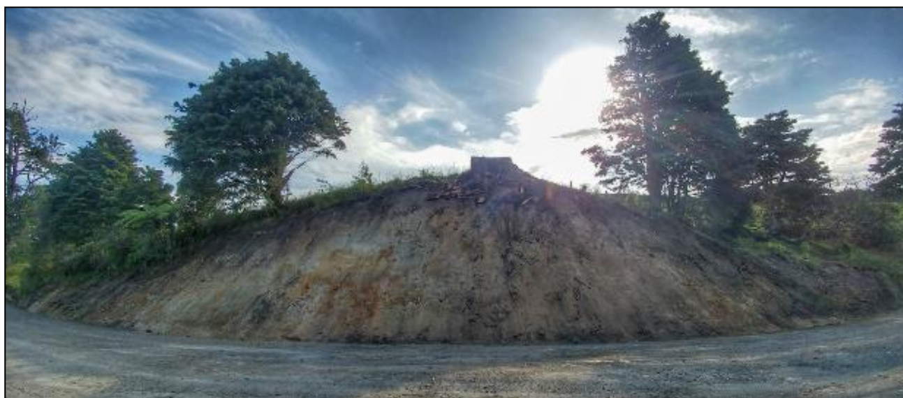
Sight improvement works – Kirikopuni Valley Road
